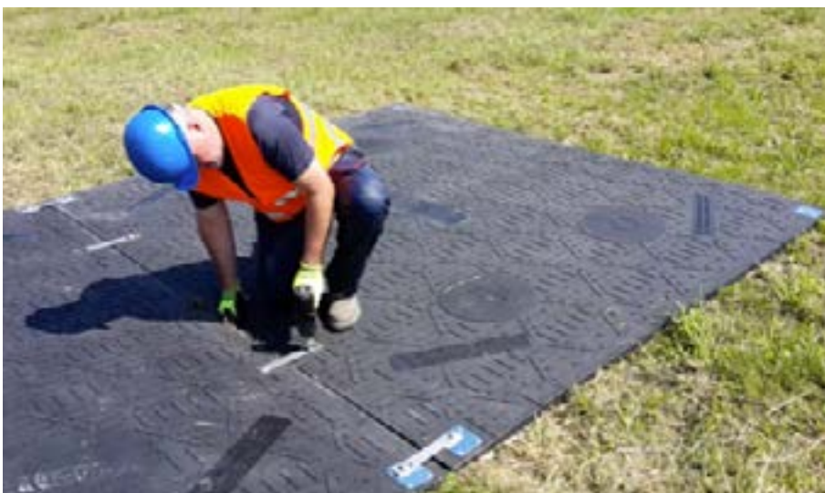
Bolts are inserted and tightened as described above for Corner Connection
