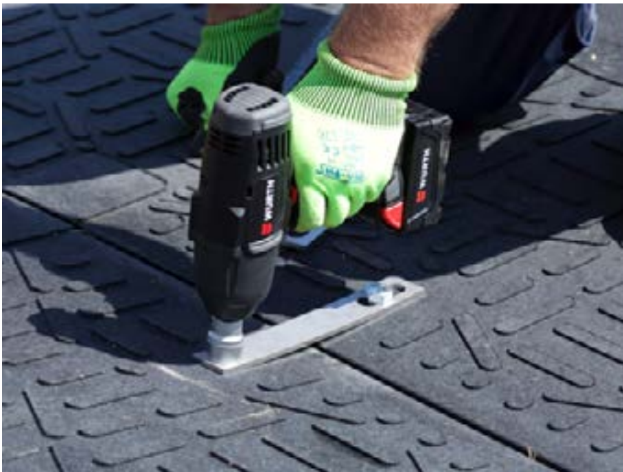
Bolts are inserted and tightened as described above for Corner Connection
