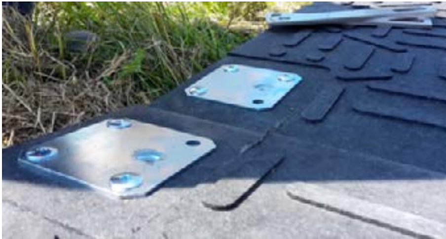
1. Adjacent mats installed ready for connection.
